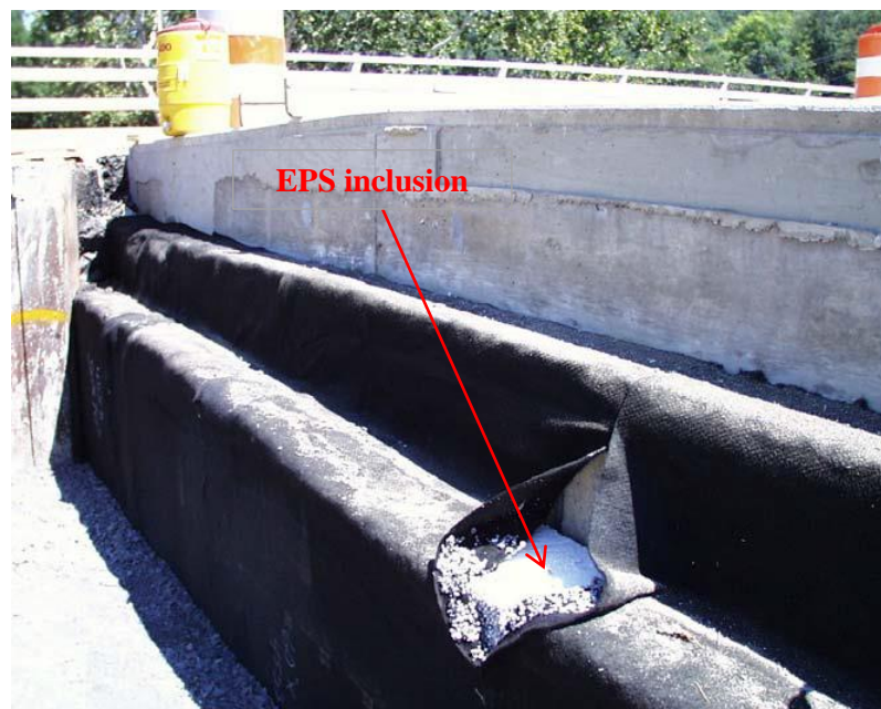
Fig. 2.20 EPS inclusion in Jackson River Bridge, Virginia, US (Hoppe, 2005)
