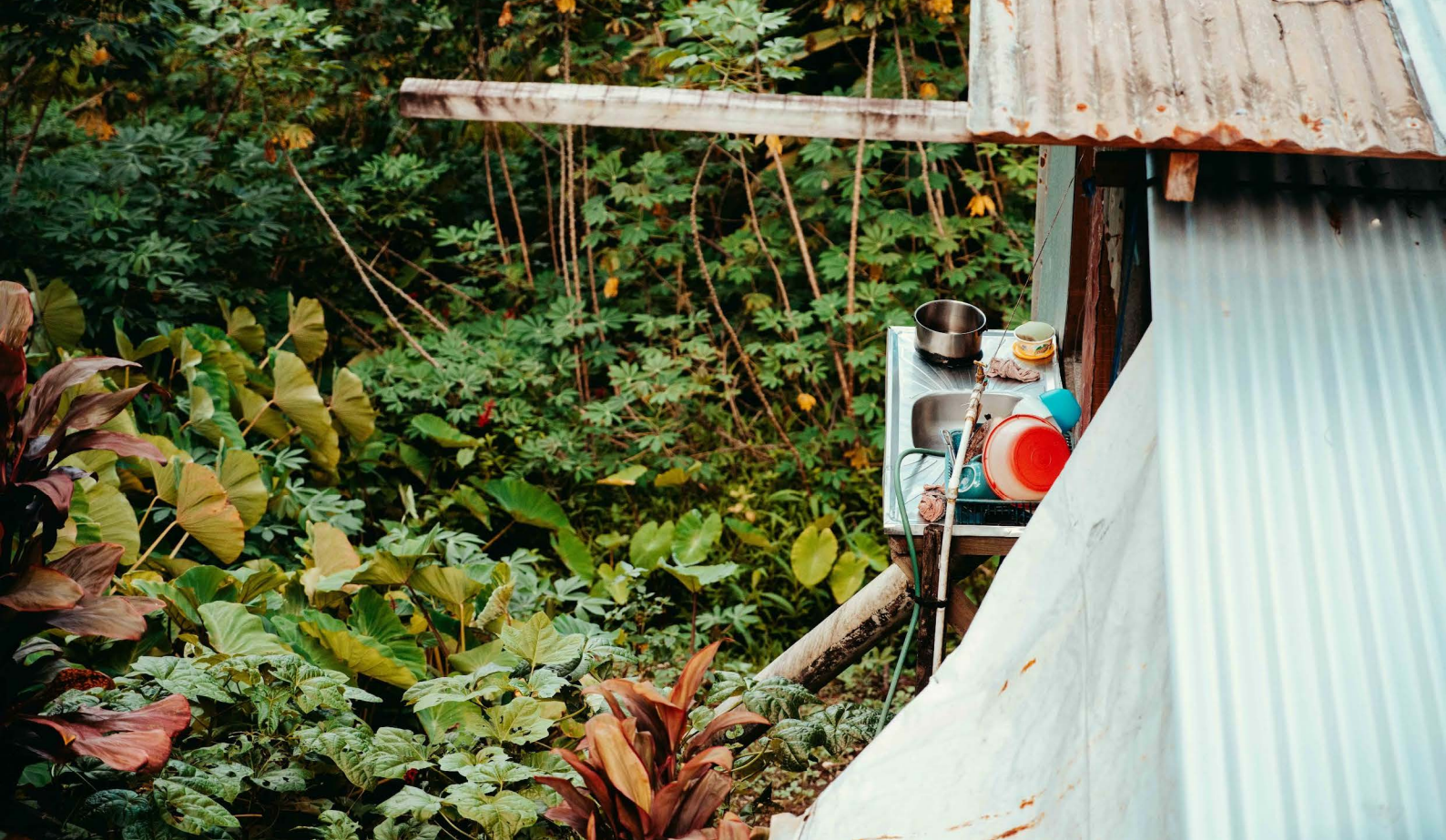
Figure 1: A kitchen sink is cantilevered from a window in Suva, Fiji. The water supply pipe is a thin, vulnerable polypipe, and wastewater is piped onto a plantation area below. (RISE program)
